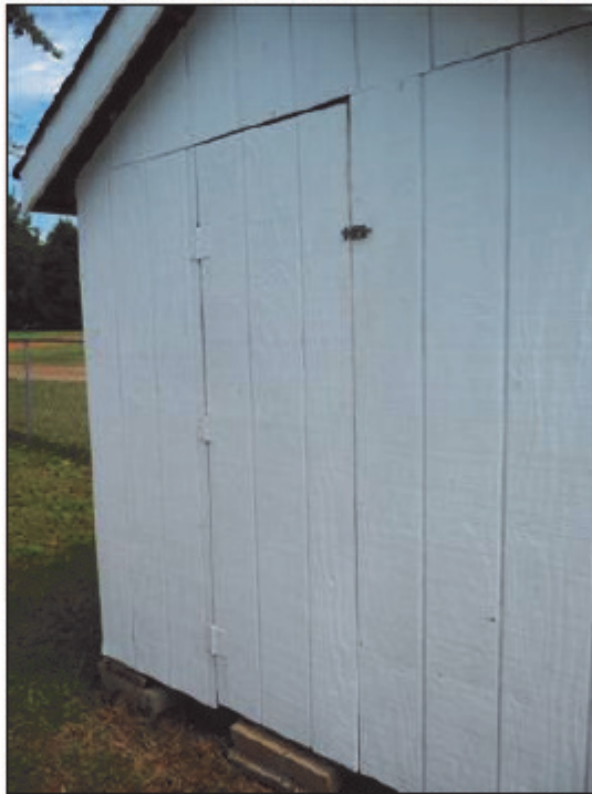
11.9 Picture 1 Shed housing pump, filter and chemicals.
