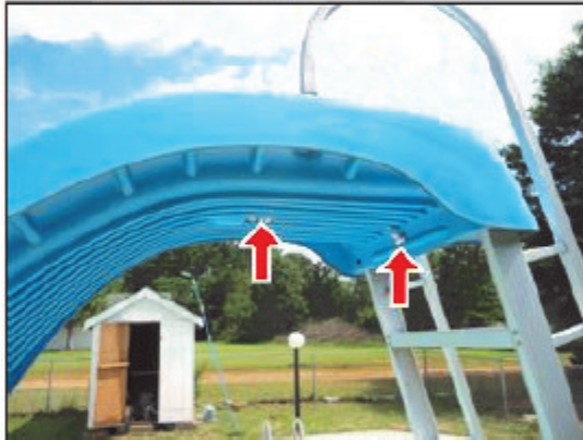
11.3 Picture 1 Water hose to slide is broken.
